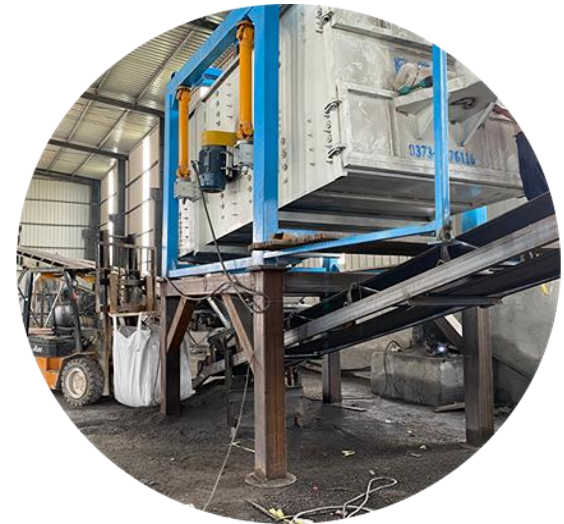
Building materials industry
